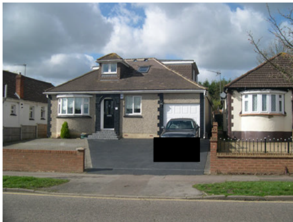
View of the front of 18 Theobalds Road.
