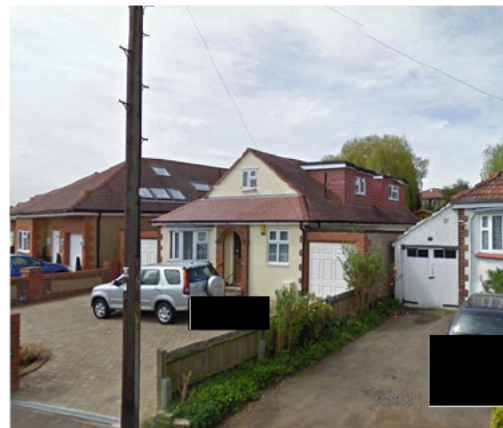
View of the dormer to roof of 30 Theobalds Road.
