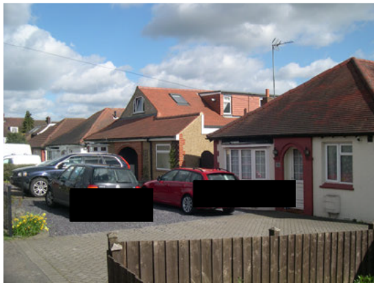
View of the dormer to roof of 17 Theobalds Road.
