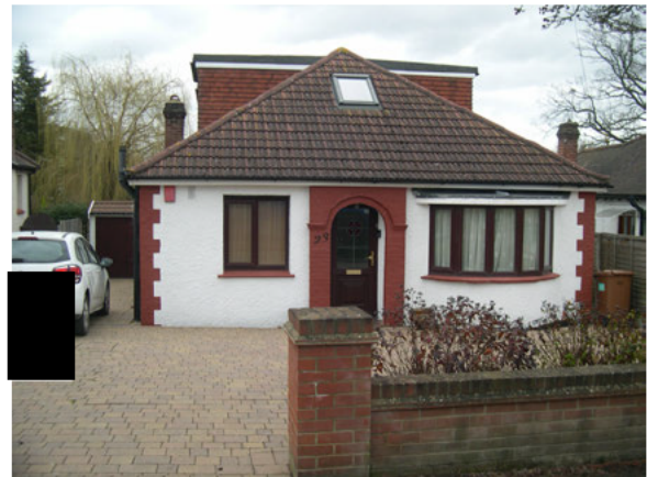
View of the front of 23 Theobalds Road
