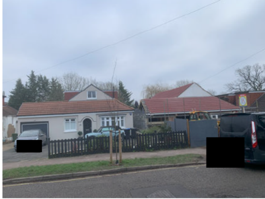
View of the front of 21 Theobalds Road behind hoarding and showing dormers to roofs of 19 and 23 Theobalds Road.
