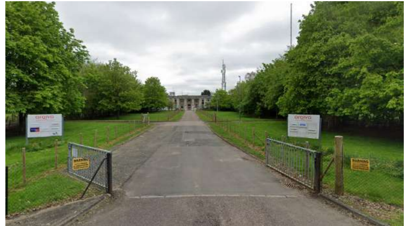
Figure 4.0 : Site access to Main Entrance road
