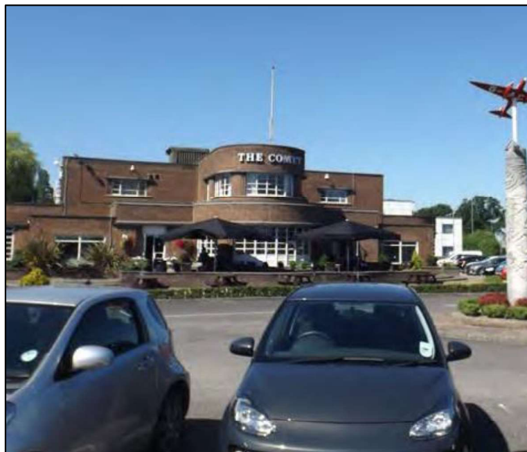
Figure 2 – Front elevation, prior to conversion/redevelopment works. Note 'The Comet' signage at first floor level.
