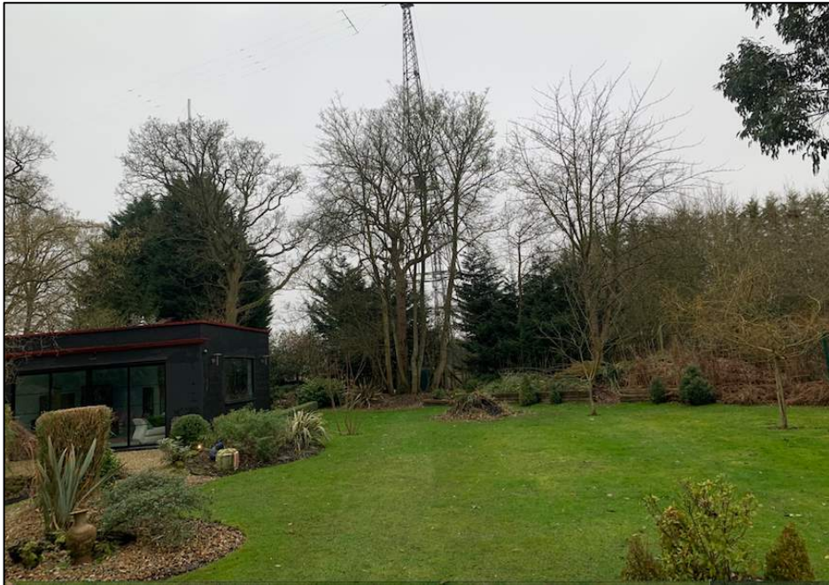
Figure 5: Photograph of Outbuilding 2 and land adjacent where the extension to the outbuilding has been erected. One of the large pylons at the Brookmans Park transmitting station is also visible.
