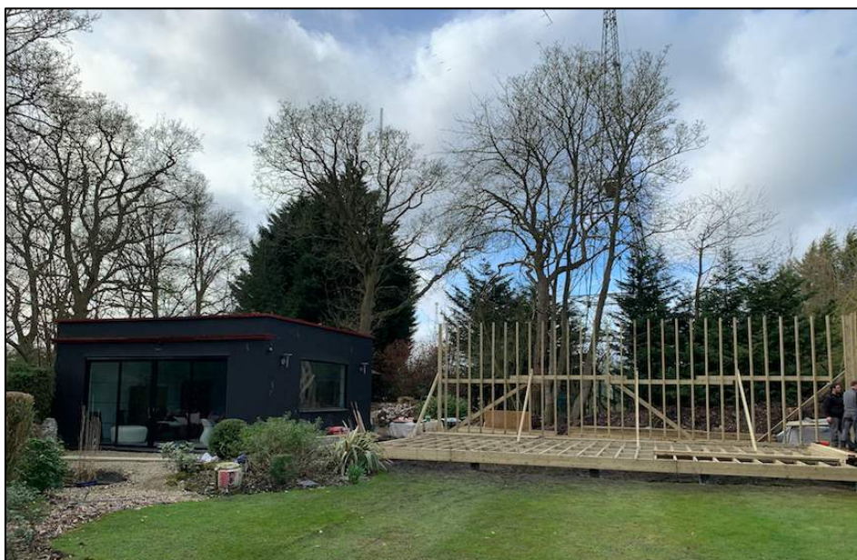
Figure 6: Construction of new outbuilding on land adjacent to Outbuilding 2
