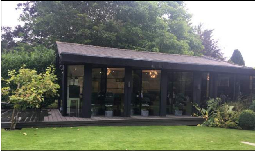
Figure 3: Photograph of Outbuilding 1
