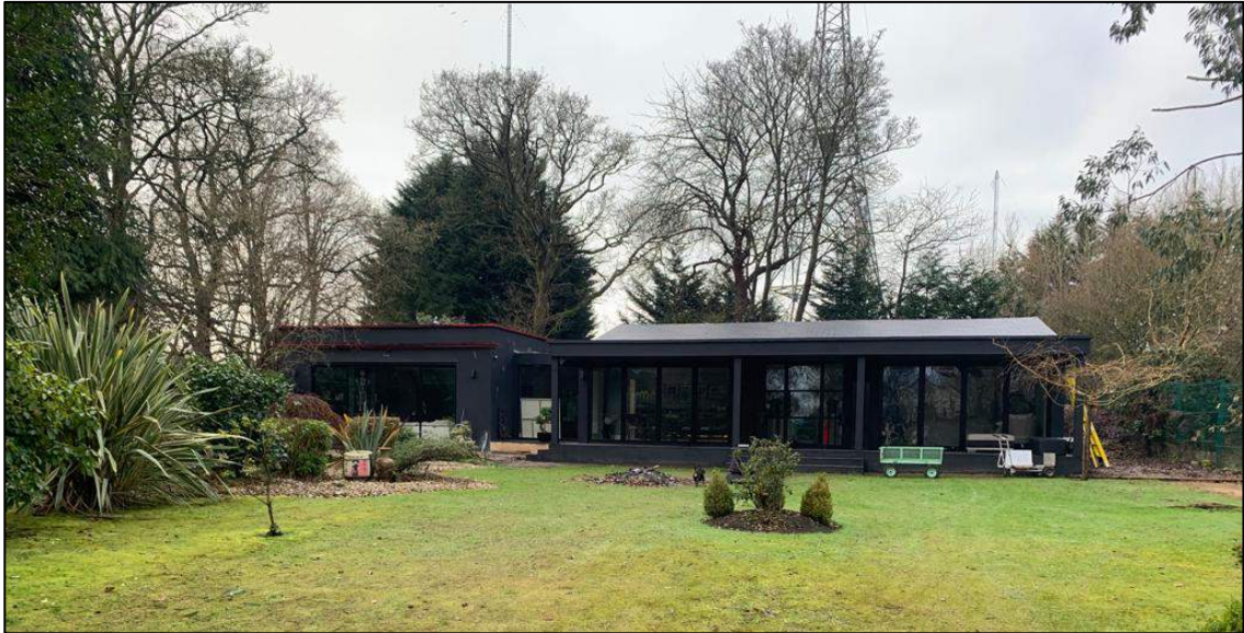
Figure 7: New outbuilding as built, connected to Outbuilding 2
