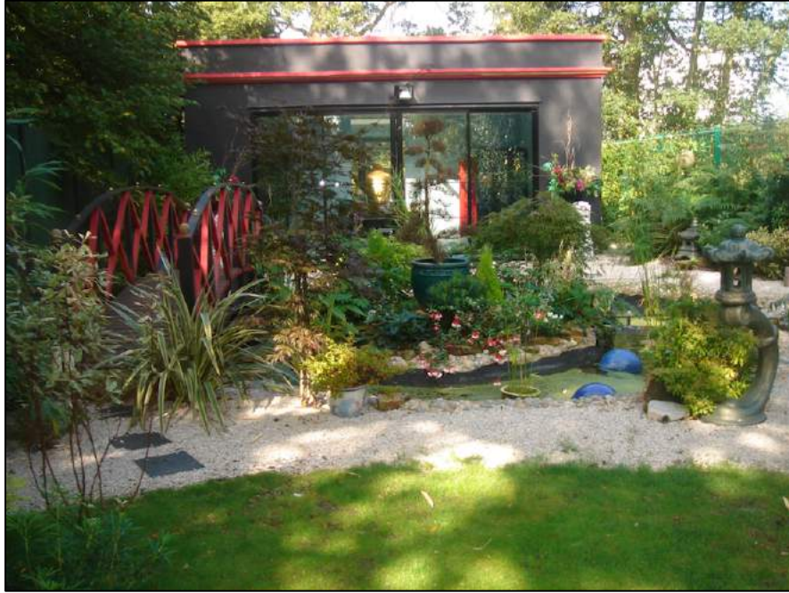
Figure 4: Photograph of Outbuilding 2 taken in 2006. NB - at this time, the Appellant's rear garden was smaller in size. The Appellant subsequently purchased an additional strip of land from the neighbouring residential property at No.53 Kentish Lane to enlarge the rear garden.
