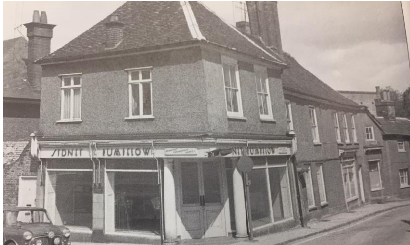
Figure 7 – Historic image (no 2) showing sashes in openings 1 & 2, a doorway in opening 3 and a sash in opening 4
