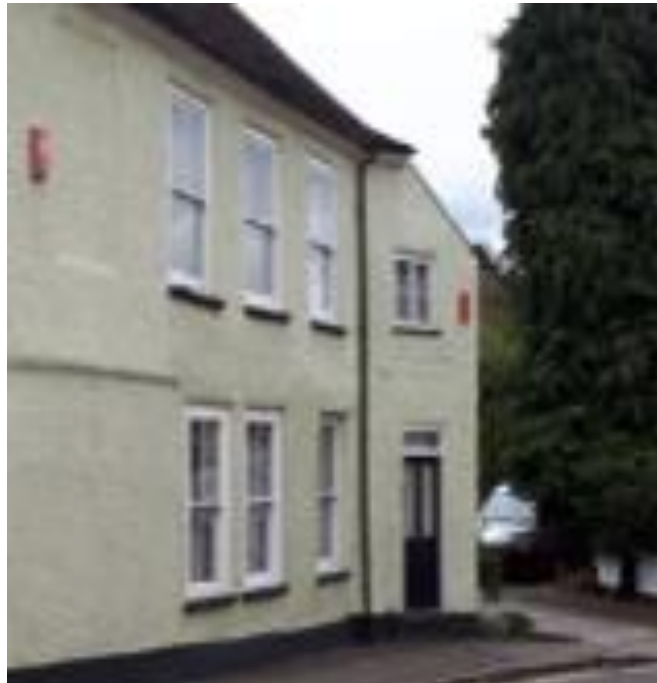
Figure 5 – Current view of the front of the property in question
