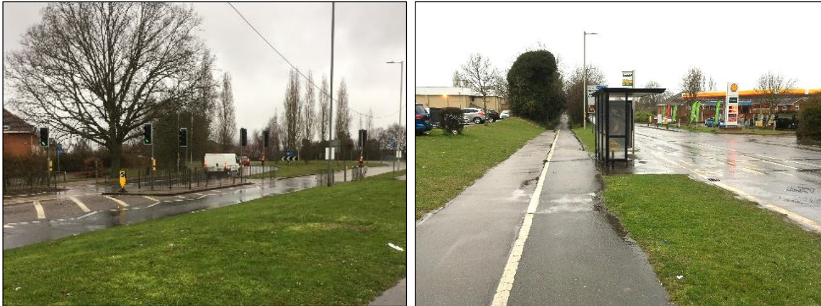
Photographs 3 & 4. Pedestrian Crossing and Footways on Stanborough Road
