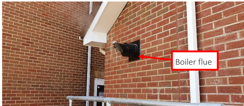
Figure 2-2 Boiler flue
