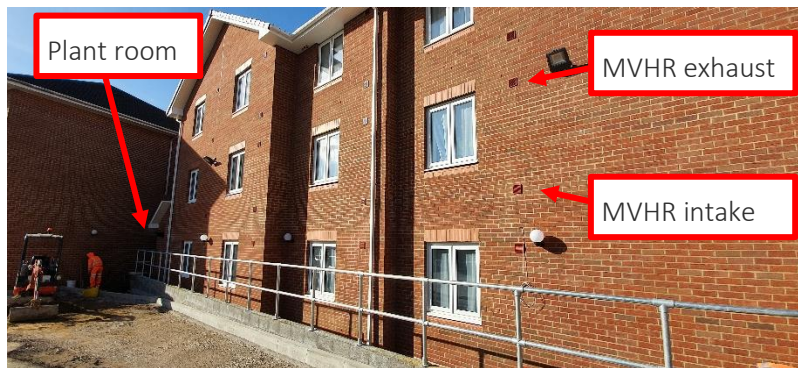
Figure 2-1 MVHR vents in south-east facade
