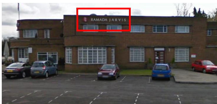
Image 7 - Existing Ramada Sign
