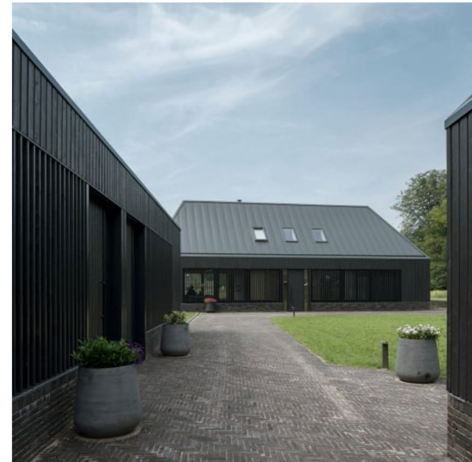
Blue-black concrete permeable paving
