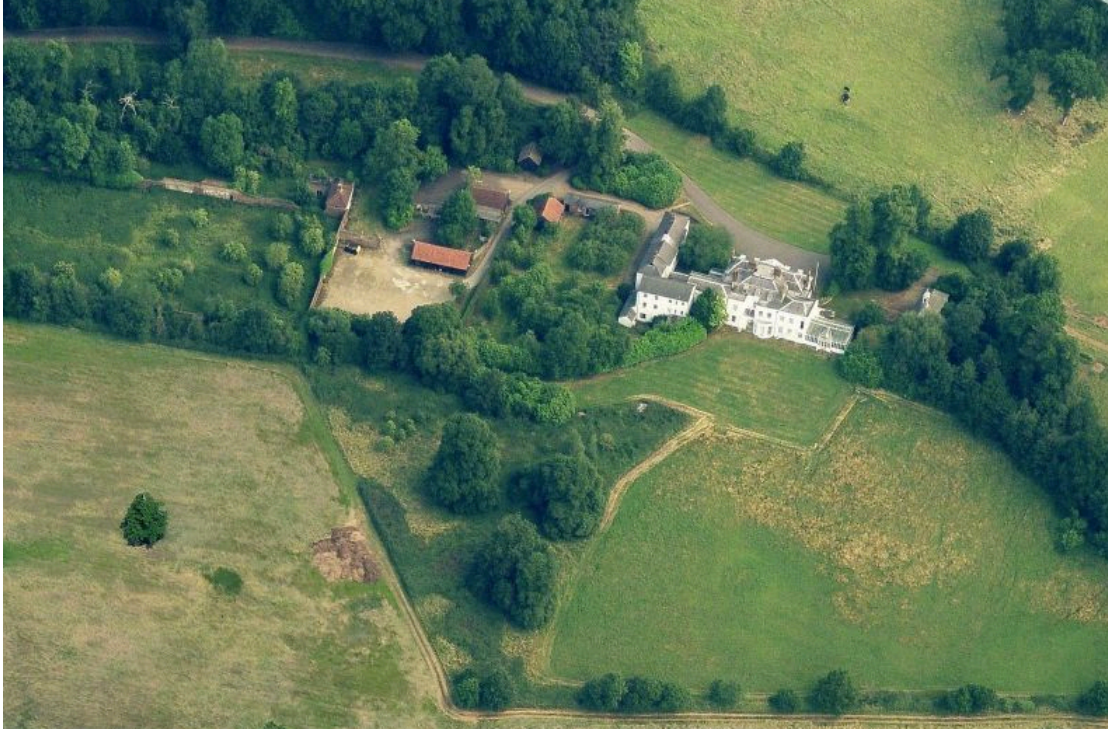
Aerial View – Northaw House
