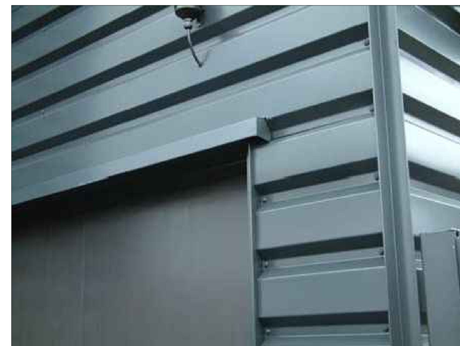
INVERTED CORNER FLASHING DETAIL
