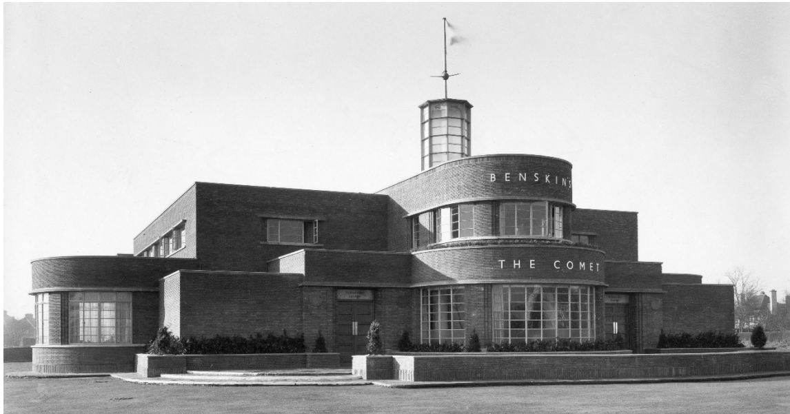
Figure 1 – 1937 photograph showing historic timber doors and blocks where the later windows (GW7, 8, 12 and 13) were inserted.
