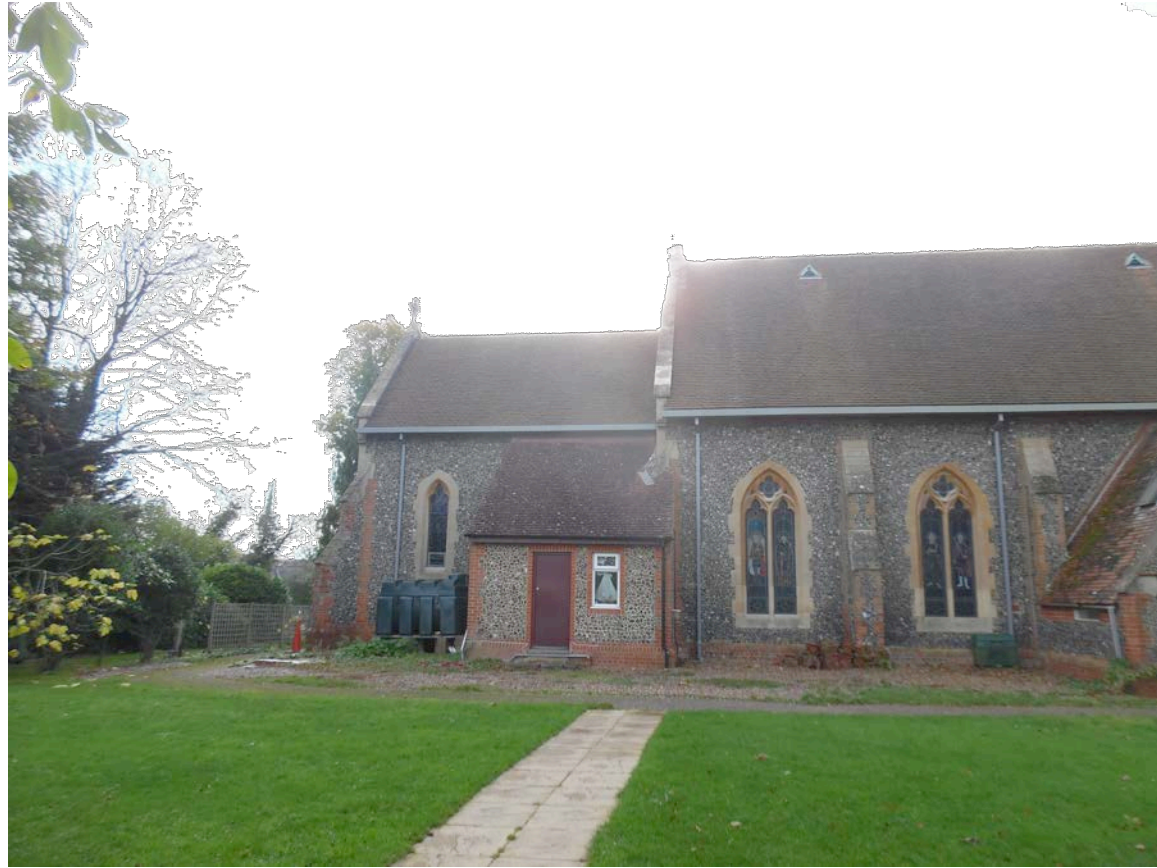
PH1 - Exterior View showing the Hall/Altar
