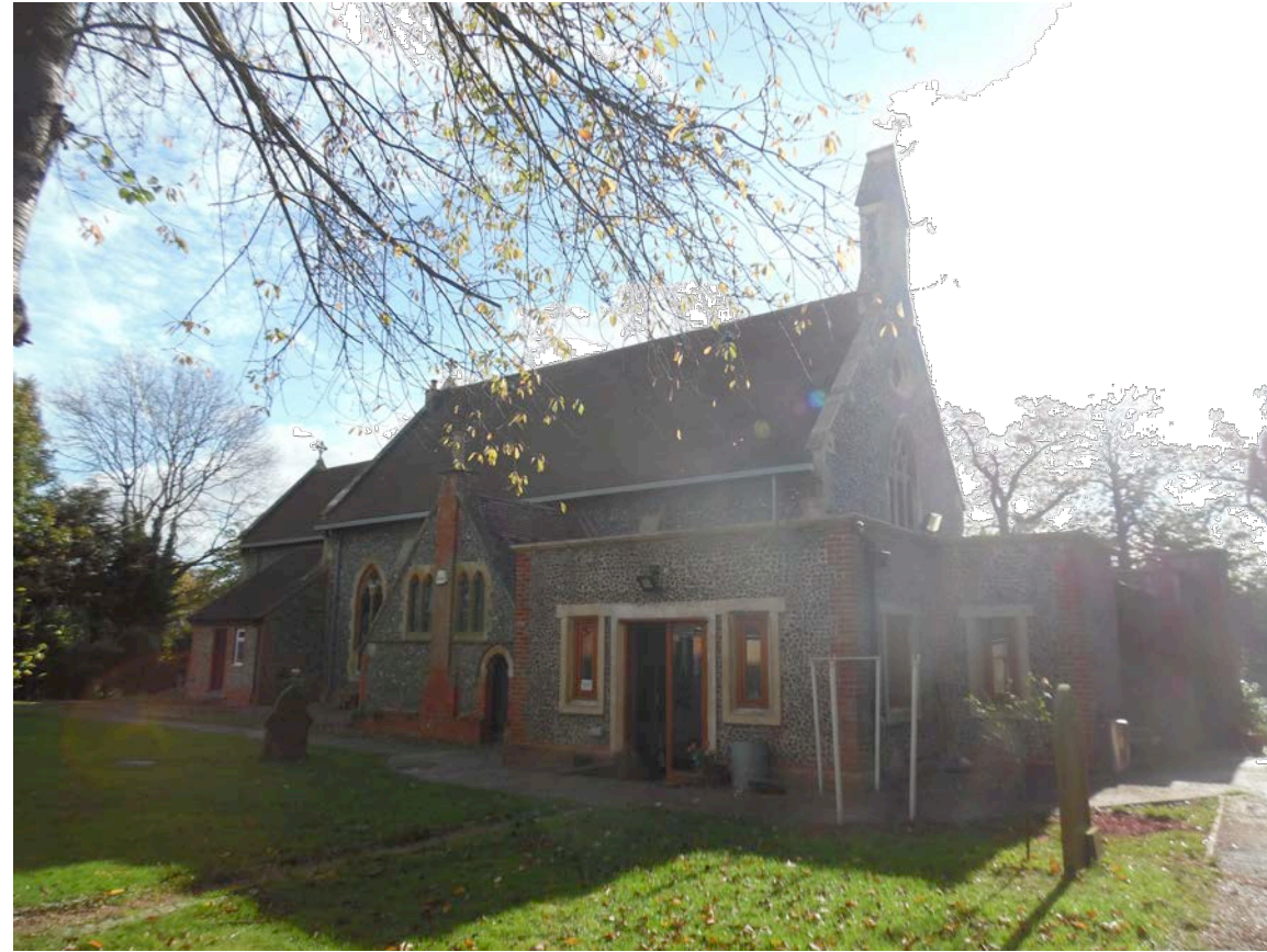
PH2 - Exterior View showing the Kitchen
