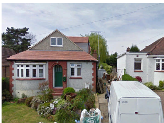
View of the front of 24 Theobalds Road.
