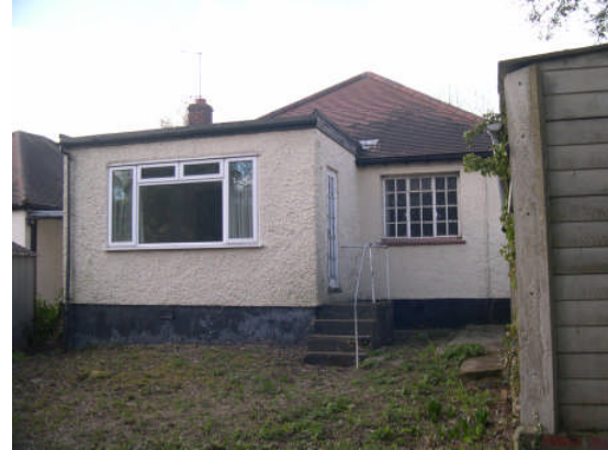
View of the rear (east) elevation from the rear garden.
