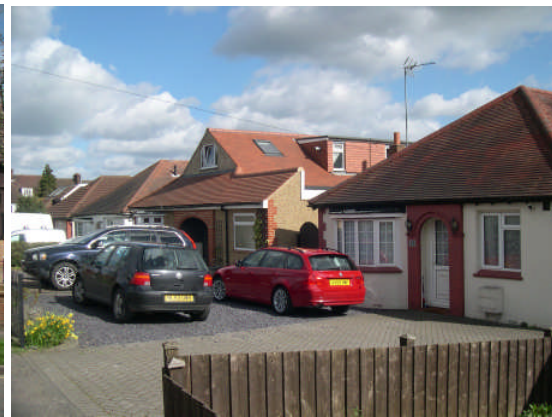
View of the front of 11 Theobalds Road
