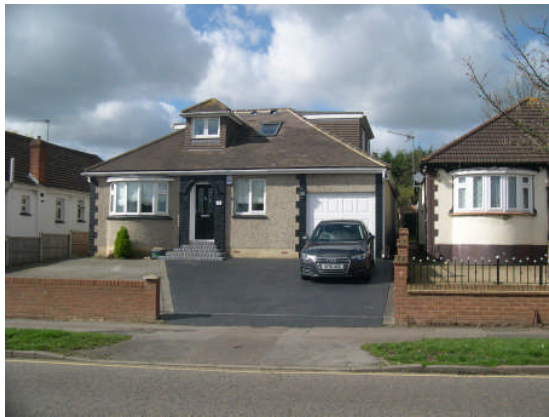
View of the front of 18 Theobalds Road.
