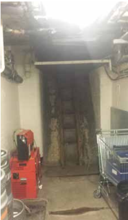
Access to basement
