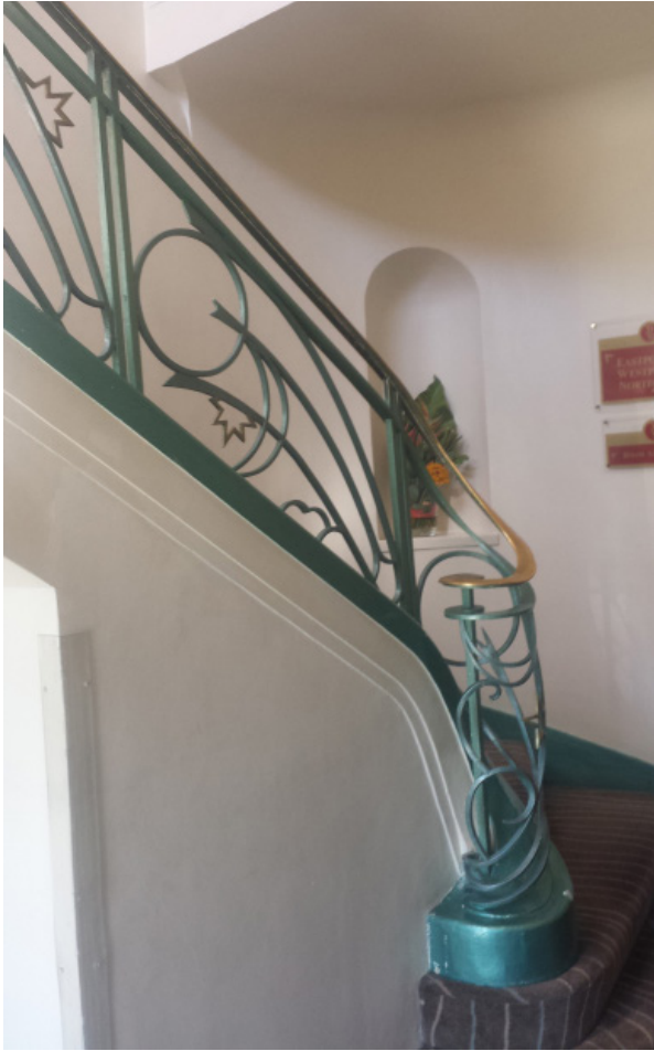
Original stair is still in situ, although the original phone box, located underneath has, at some date, been removed.
