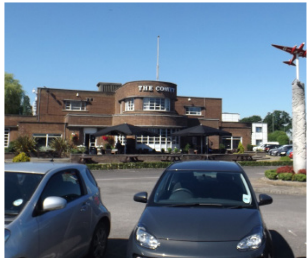
Externally the building has had a number of unsympathetic alterations in terms of addition signage, lights and repair work.
