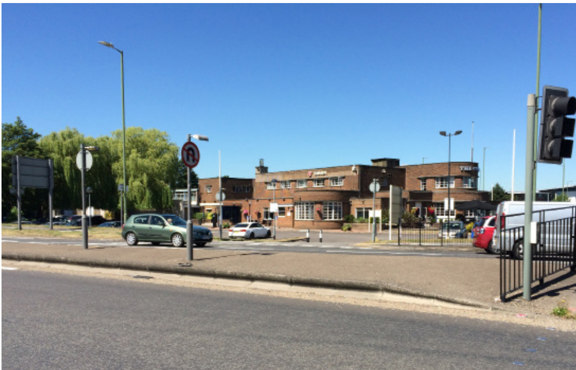
The view westwards from Comet Way towards the front (north) and side (east) elevations of the Comet Hotel. Although there is some foreground intrusion caused by the highway engineering, the low form of the hotel can be made out, as can the rounded bat elements. From this viewpoint, the current condition of this setting is not beneficial and makes only a low level of contribution to significance. The scale and visual dominance of the highway engineering is harmful.
