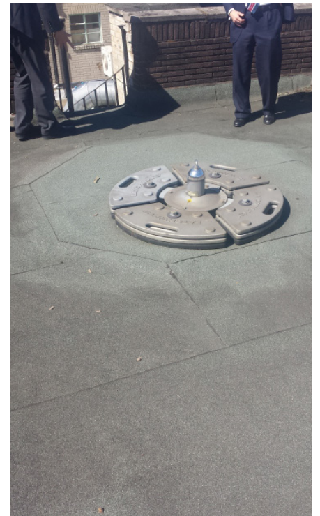
Opening in roof for original lantern still visible.
