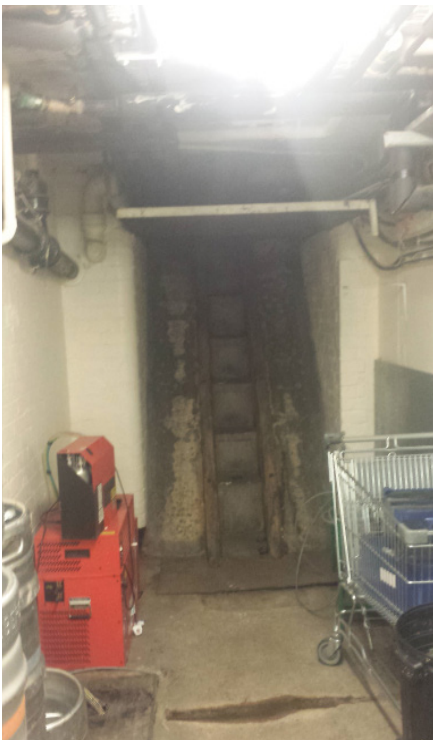
Access to basement
