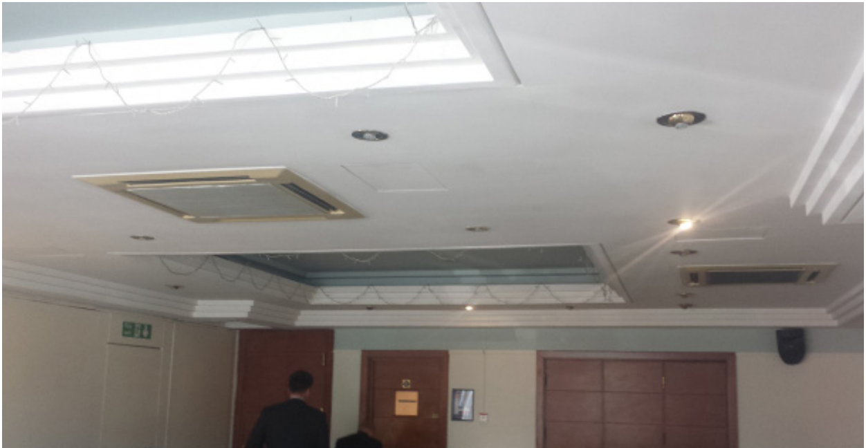
Example of lowered ceiling, installed during a previous refit (prior to listing). Above the suspended ceiling, all trace of former finishes has been removed.
