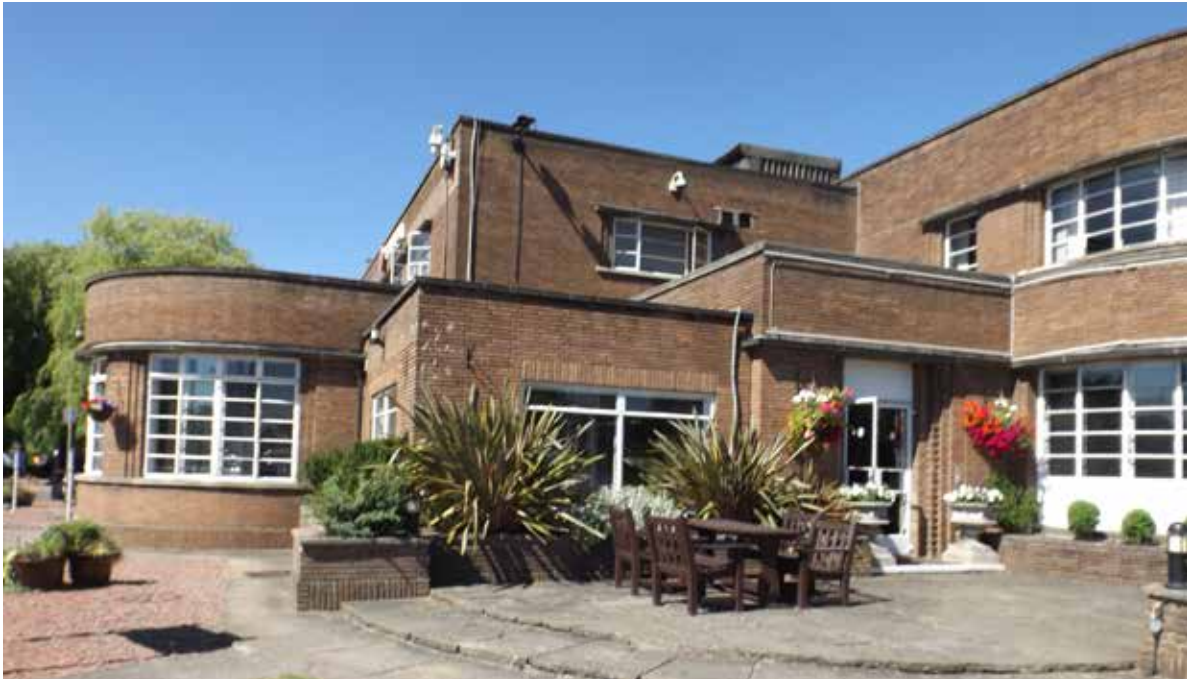
Side elevation of the Comet Hotel
