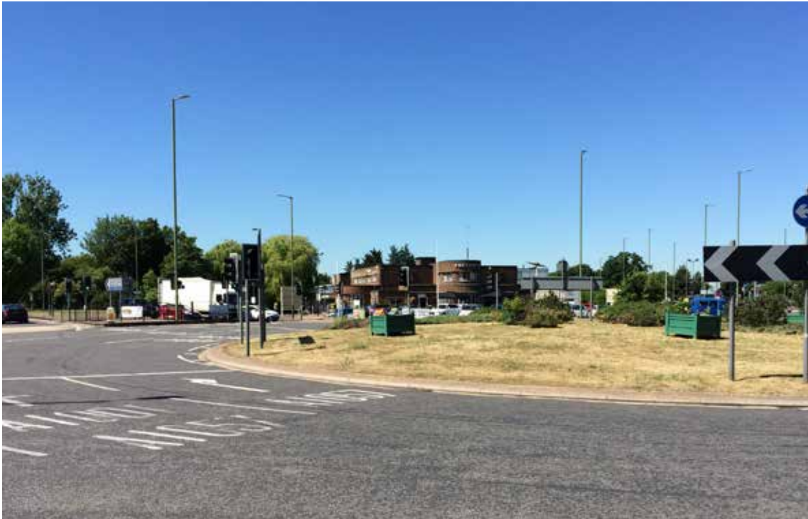
The view south-westwards from Comet Way across the roundabout at the junction with St Albans Road West towards the Comet Hotel. Due to the building's relatively low level and emphasis, it does not perform a strong landmarking role at this distance, particularly in view of the foreground road surfaces, signage and lighting columns. Contribution of this setting to the significance of the asset is low . The scale and dominance of the highway engineering is harmful.
