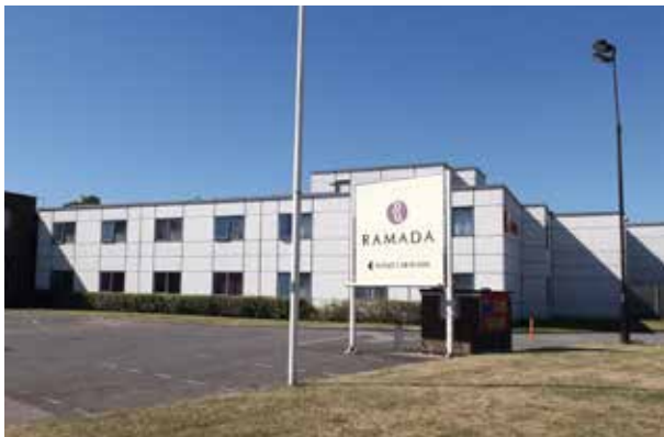
Existing hotel block accommodation
