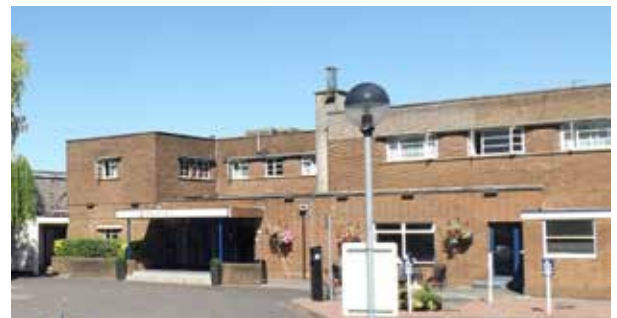
Unsympathetic extensions and additions have been added over time including a small extension to the side of the main bar, and the infilling of the rear courtyard and creation of the reception area.
