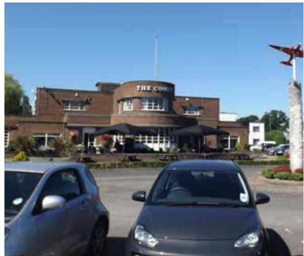
Externally the building has had a number of unsympathetic alterations in terms of addition signage, lights and repair work.
