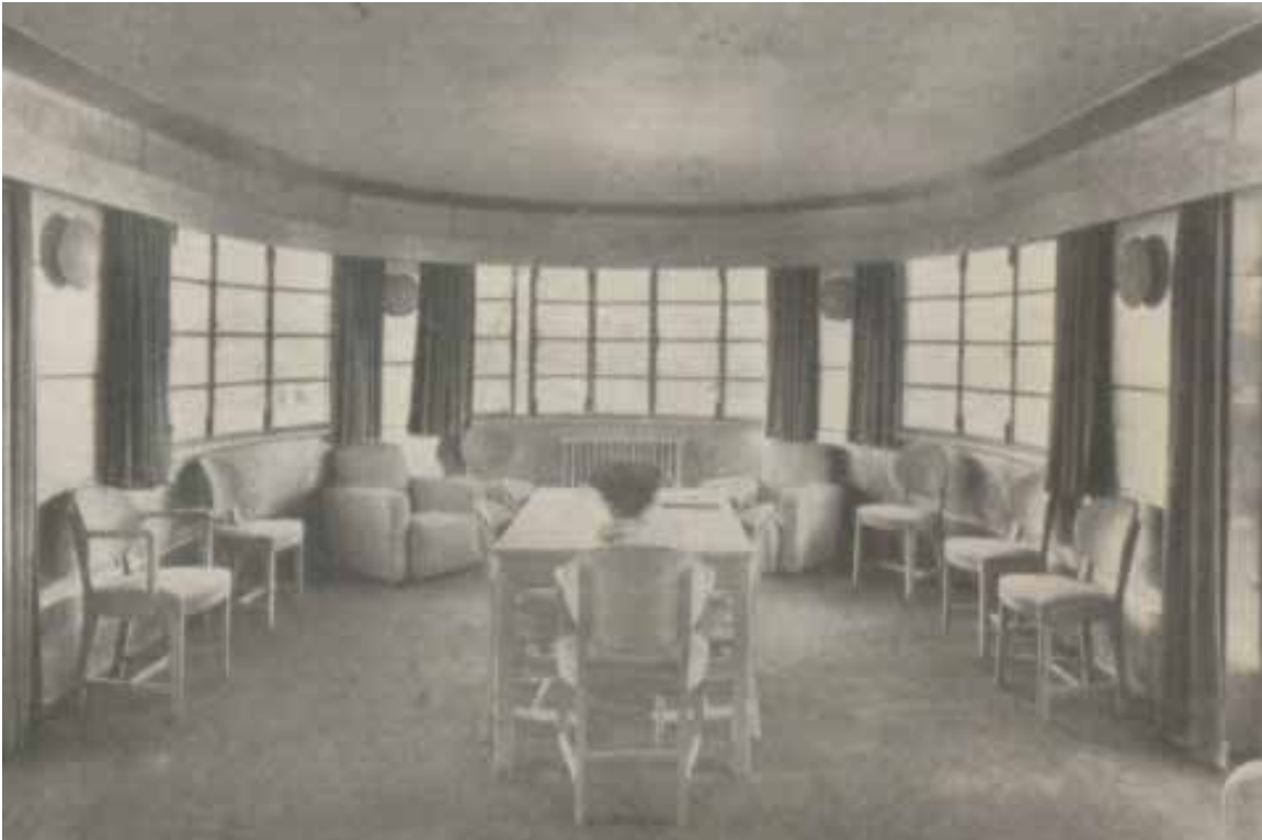
The first floor Sitting Room of The Comet with silver gilt panelling - taken from The Architect and Building News , January 1937, p97
