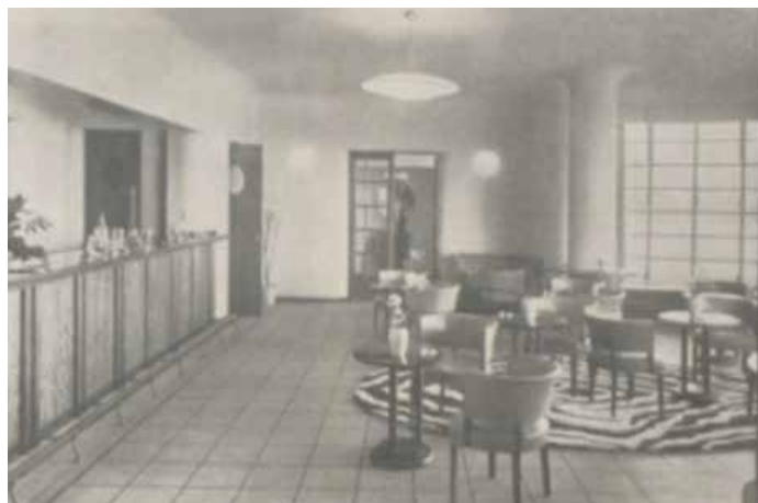
Interior of The Comet - Taken from the Architect and Building News, January 1937, p97
