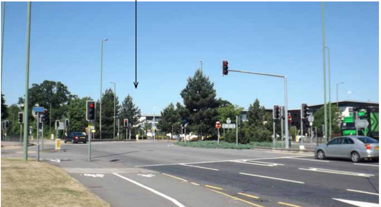
Location and setting of the milepost, which is dominated by the highway infrastructure.
