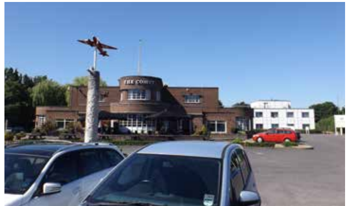
The view towards the front elevation will be improved by the reinstatement of the lantern, one of its most important original features
