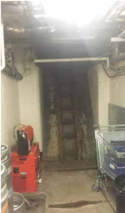
Access to basement
