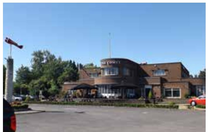
Front elevation of the Comet Hotel
