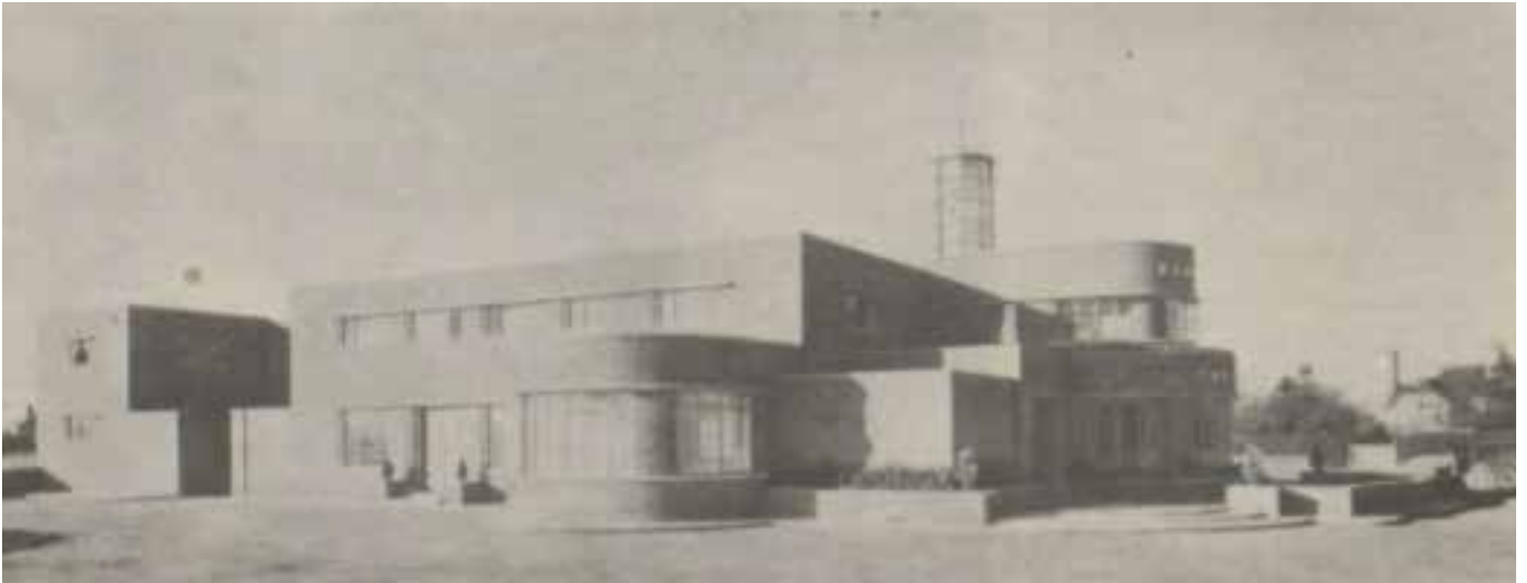
The Comet: the roof is used to watch air displays - Taken from The Architect and Building News, January 1937, p94
