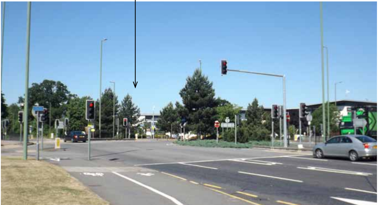
Location and setting of the milepost, which is dominated by the highway infrastructure.
