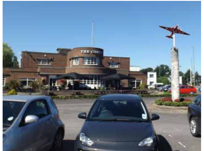
Externally the building has had a number of unsympathetic alterations in terms of addition signage, lights and repair work.
