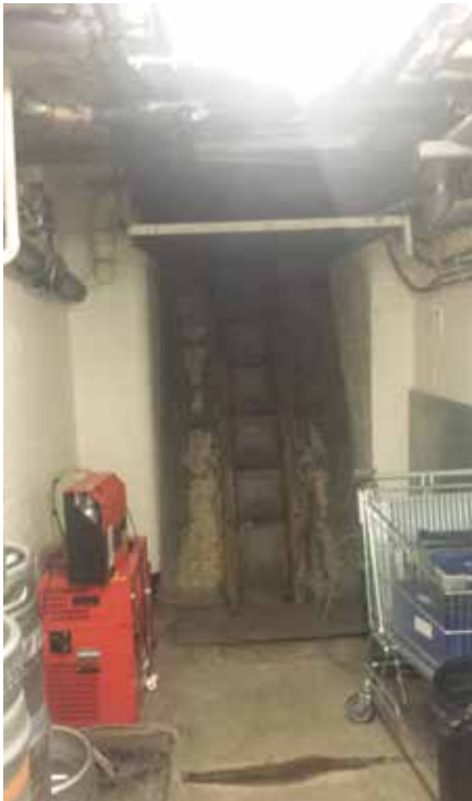
Access to basement
