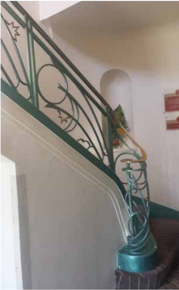
Original stair is still in situ, although the original phone box, located underneath has, at some date, been removed.
