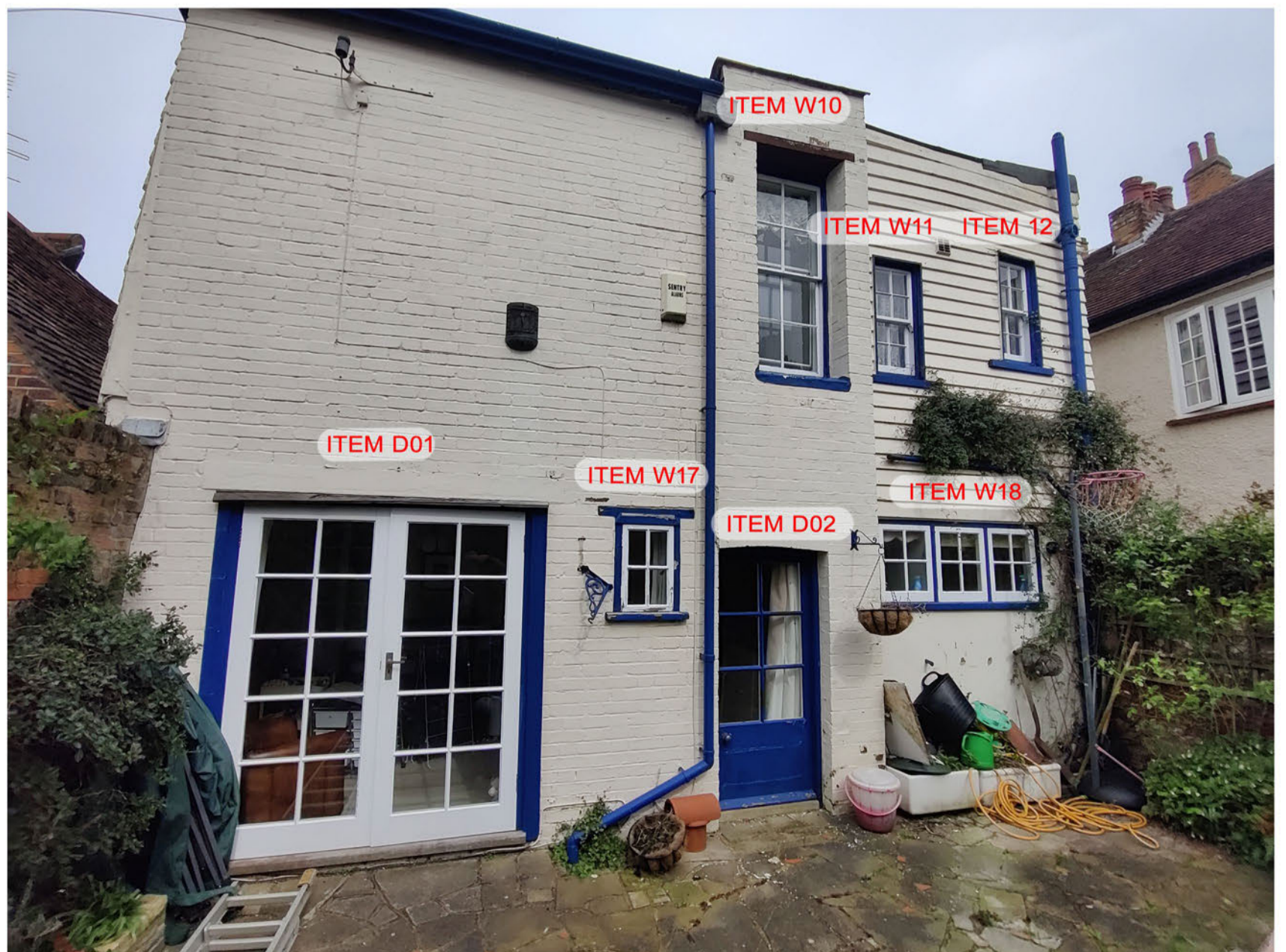
Rear elevation of house
