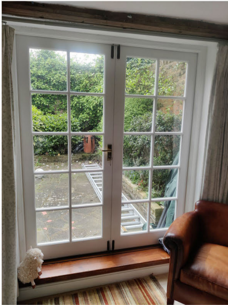
ITEM D01 - FRENCH DOORS OPENING OUT. NEW DOOR LEAVES ARE NOT PRACTICAL TO FIT TO EXISTING FRAME, AS HARD TO WEATHERSEAL AND LOCK SECURELY. COMPLETE NEW DOORS TO BE FITTED. GLAZING PATTERN TO MATCH EXISTING. CURRENT GLAZING BARS ARE 25mm WIDE, NEW TO BE 24mm WIDE. CURRENT GLAZING IS SINGLE GLAZED. NEW DOUBLE GLAZED WITH A SLIMLINE WHITE SPACER. PAINTED WHITE SASHES EXTERNALLY WITH ALL FRAMES AND CILL BLUE AS EXISTING.
