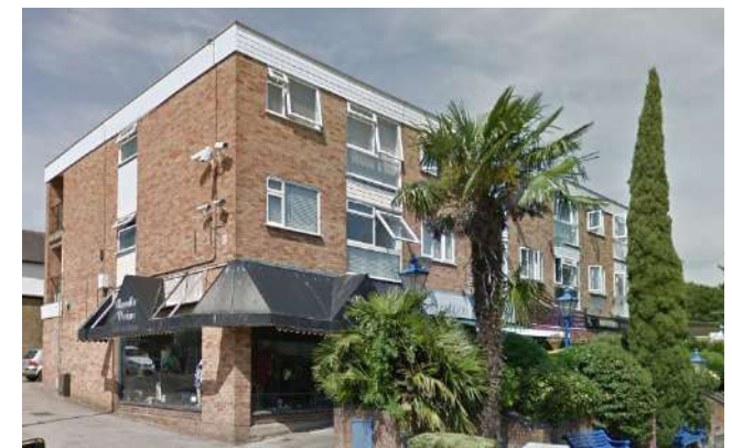
View of the Site from corner of Station Rd & Maynard Place
