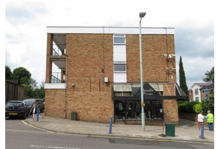
Image of the side of the of the building
