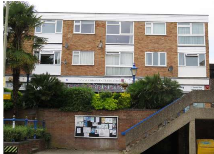
Image of the front facade
