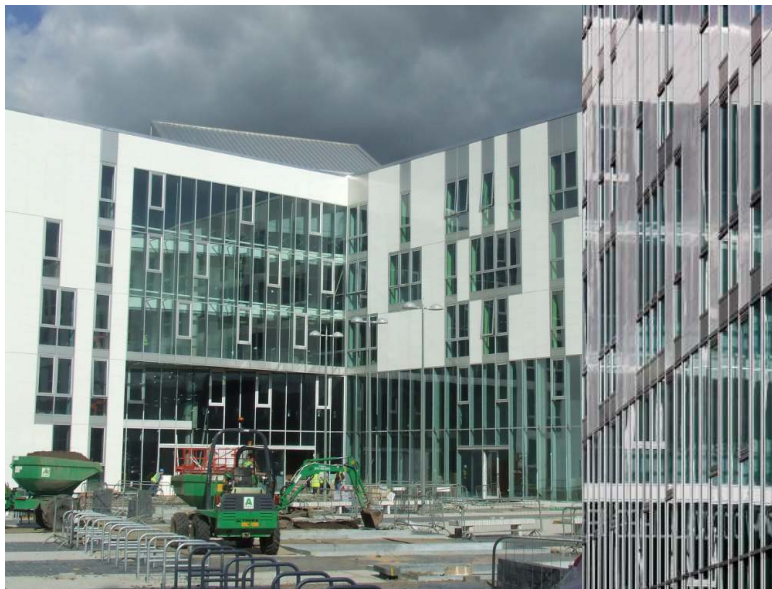
Panelled cladding system
