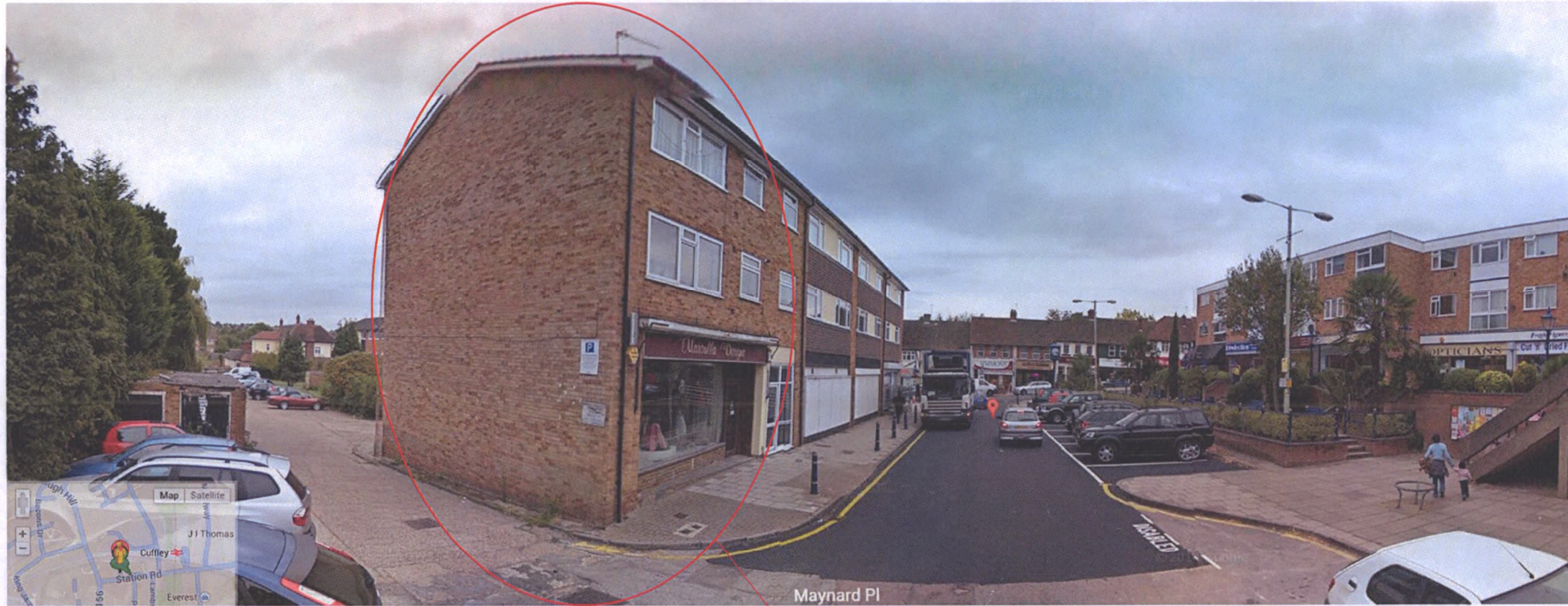
No 17 (Shop) & 17a flat above - view from Maynard Place
