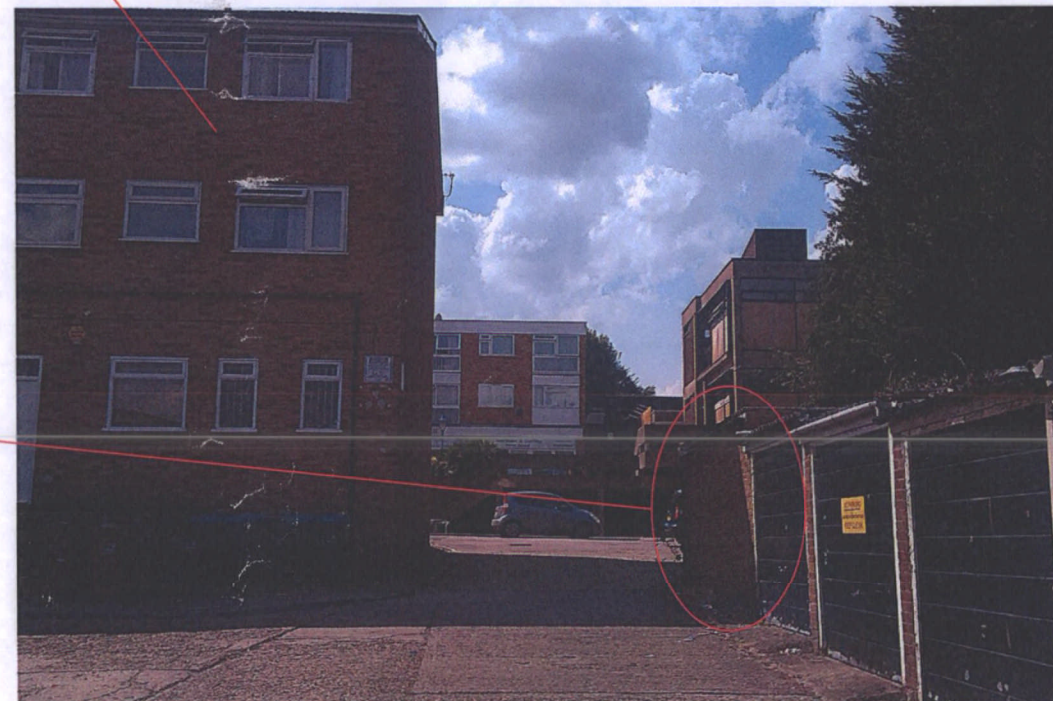
view from behind (east facing) and site shed & 2 garages
