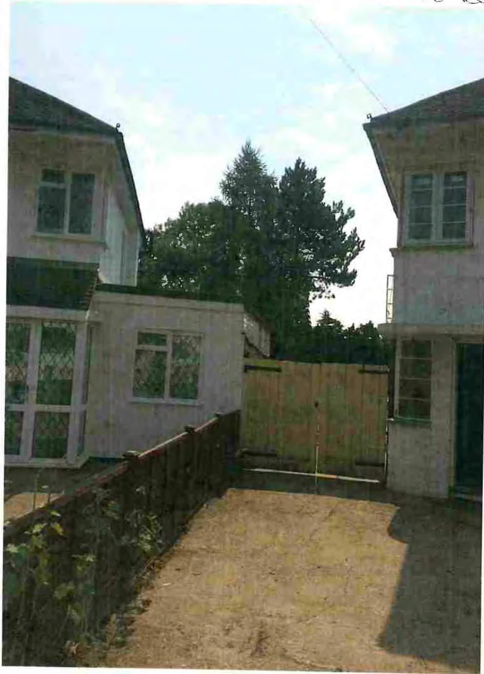
SITE FROM BRAMBE ROAD
