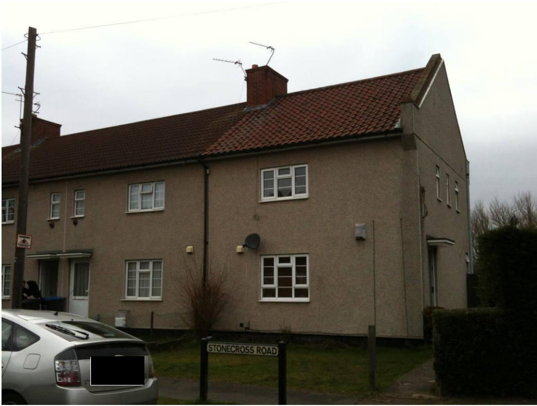
Photograph 1 – Cross Elevation of the Property
