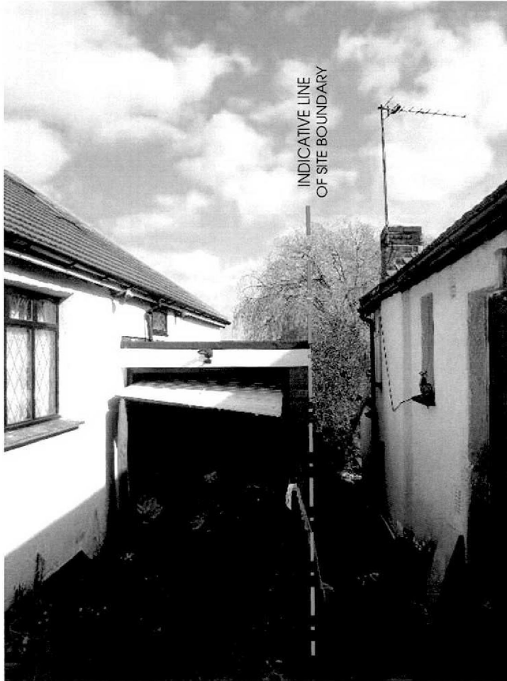
FRONT OF EXISTING GARAGE - FACING NORTHAW ROAD EAST
