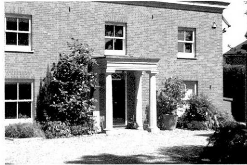
Precedent: Portland Stone portico at No 26 The Ridgeway
