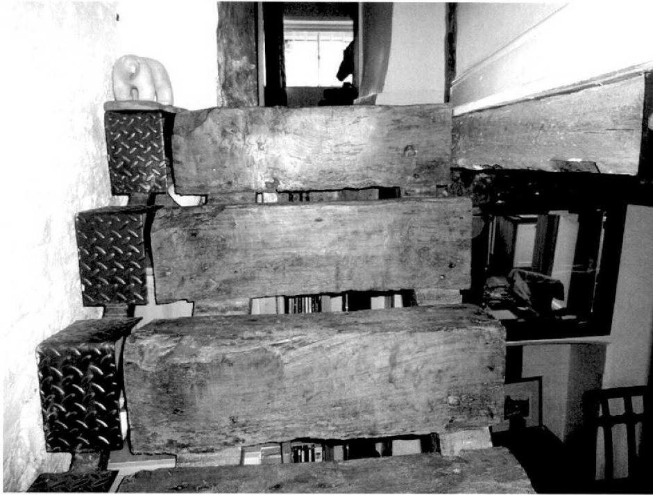
Original treads with steel make up pieces.
