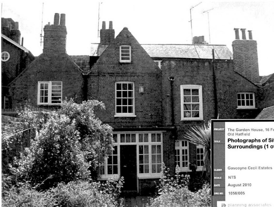
Photo 2: View of the rear of the house showing projecting gable and shallow flat roofed extension to drawing room.
