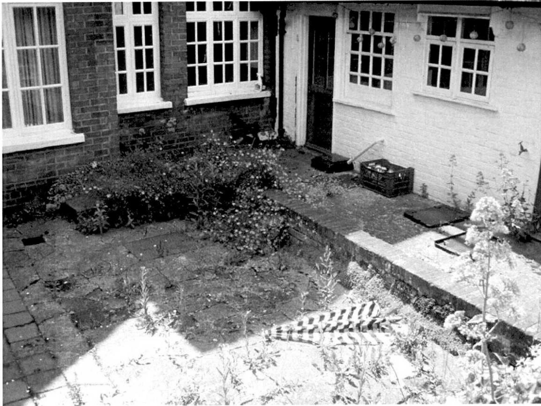
Photo 5: View of rear patio area showing position of the proposed single storey extension.
