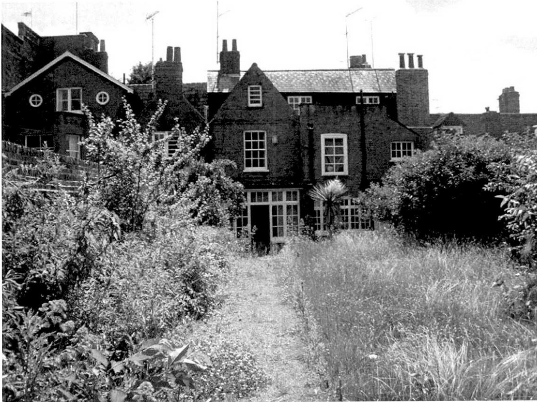
Photo 1: View of rear elevation from garden showing existing rear extensions.
