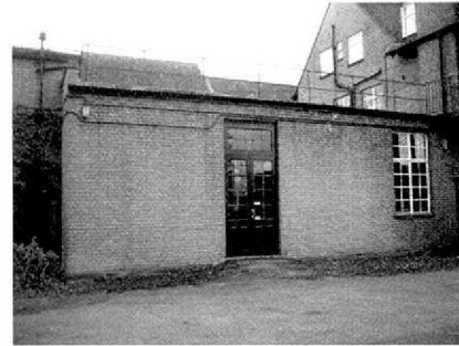
Single storey extension
