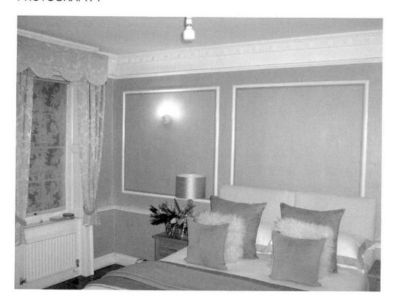
Position of doorway from Master Bedroom into Bathroom 1. The panels are formed by planted timber mouldings and are thought to be recent. The opening will be positioned to minimise loss of studs and will be framed in pine re-using the existing door frame, architraves and panel door.
